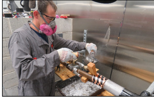
Image Courtesy of Quanta Underground
