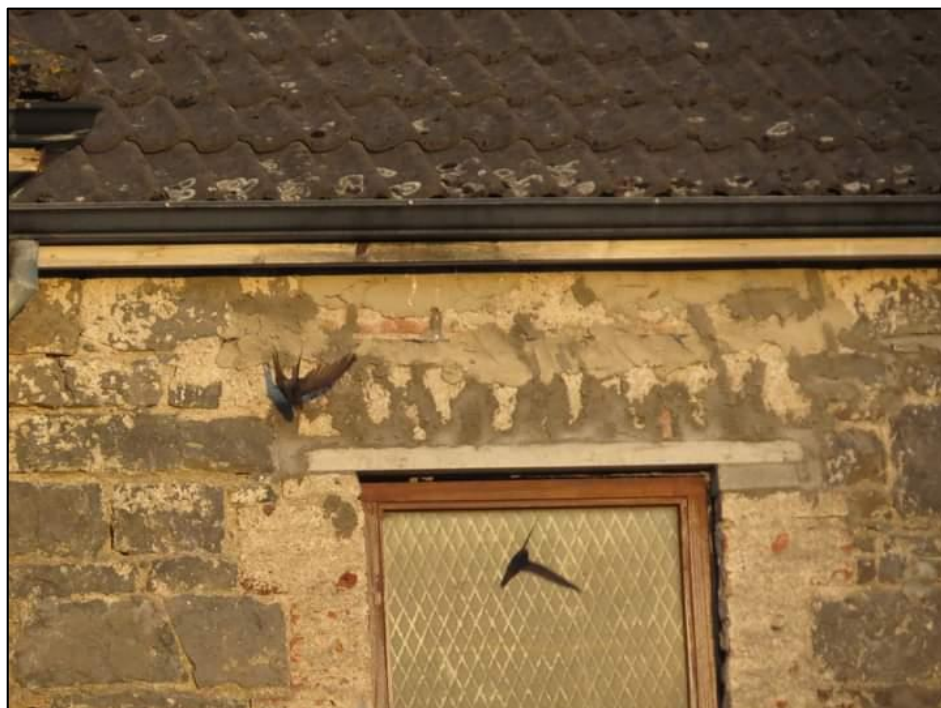
Figure 3. Swift exiting nest site from behind timber fascia as another bird passes by. (image from Carlow Youth Centre).
