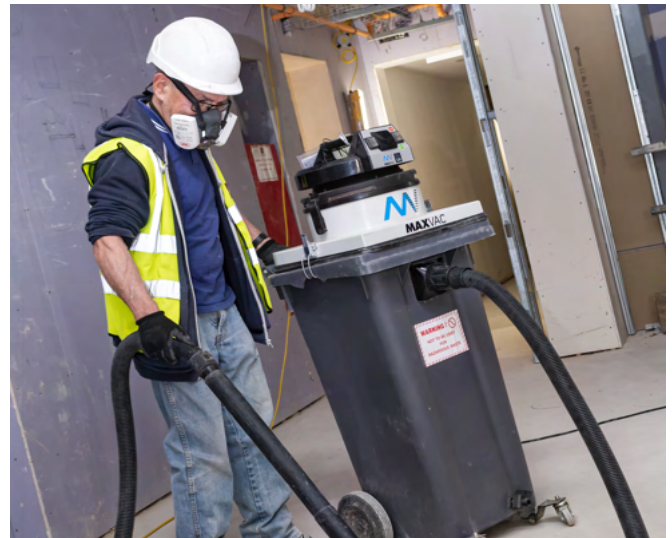
Figure 1: Half mask respirator in use.
