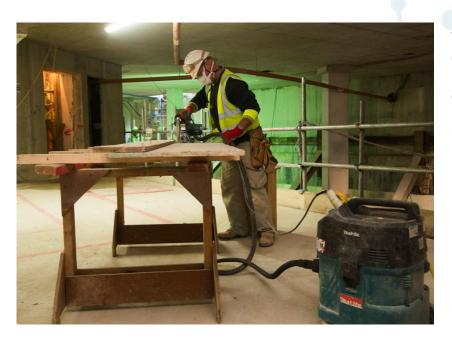
Where power tools are used on-site for wood working, dust exposure can be controlled by using local exhaust ventilation (LEV). Most commonly in construction this will involve on-tool dust extraction consisting of:
