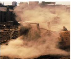
Demolition dust is commonly produced during the use of high powered grinding, scabbling and breaking demolition machinery in 'hard' or structural demolition.
