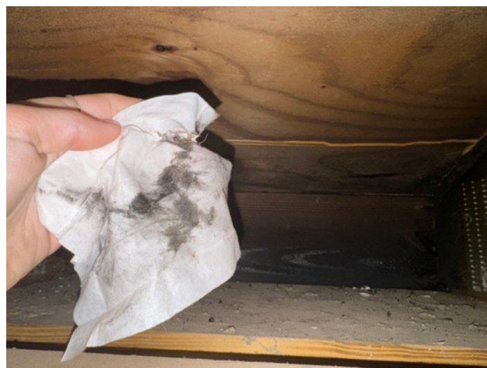
Upper Level: Soot deposition in plenum
