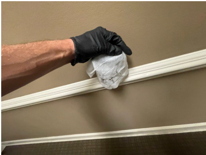
Main Level: Soot definition on surfaces.
