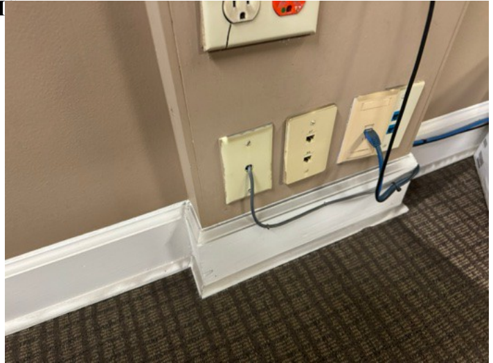
Main Level Offices: Soot on switches and outlets
