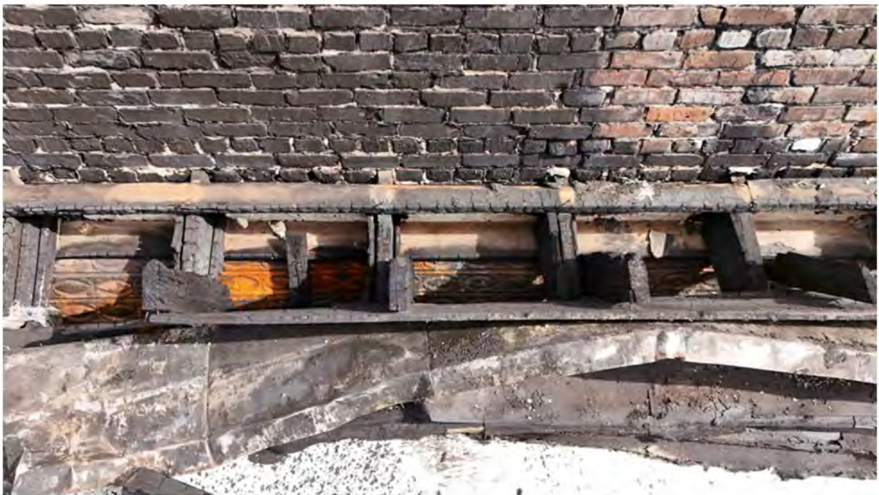
52. Charred framing from the adjacent building.
