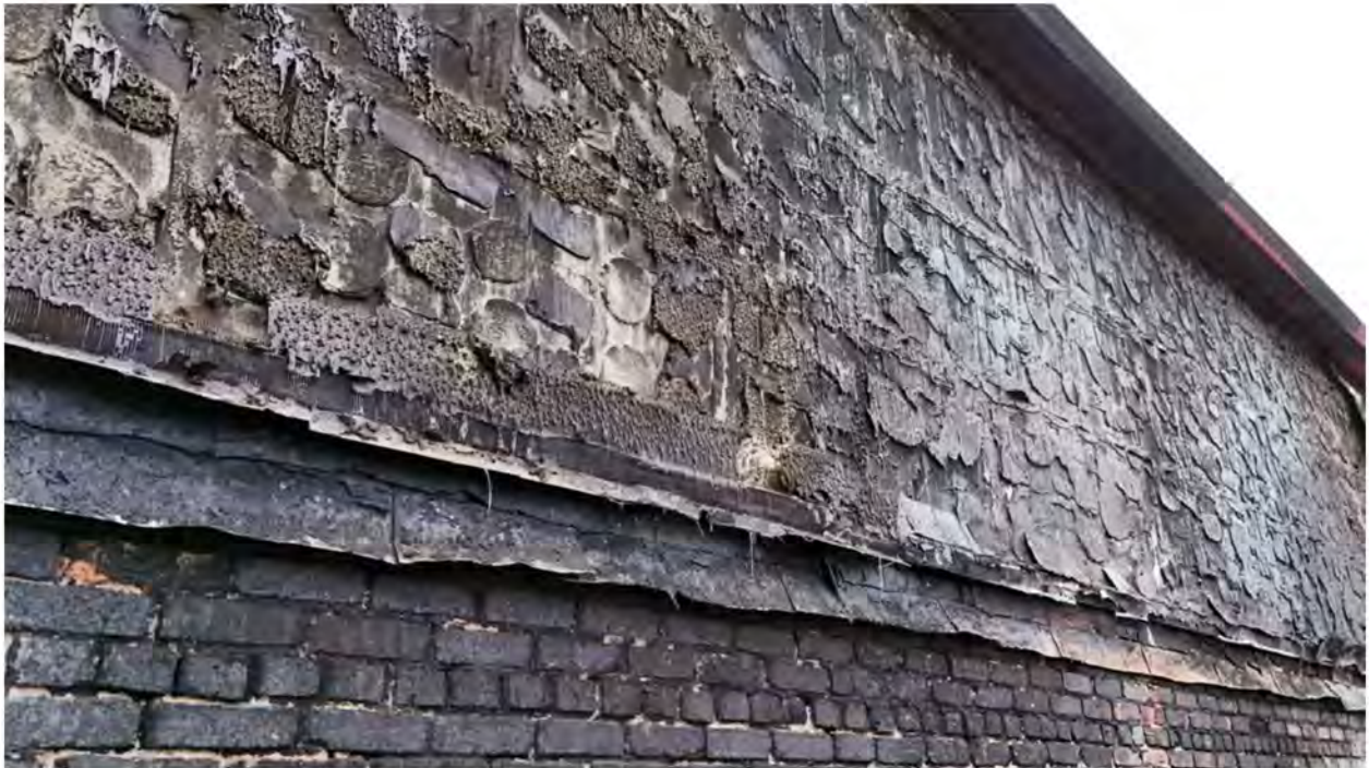
50. Flashing between the first and second floor.
