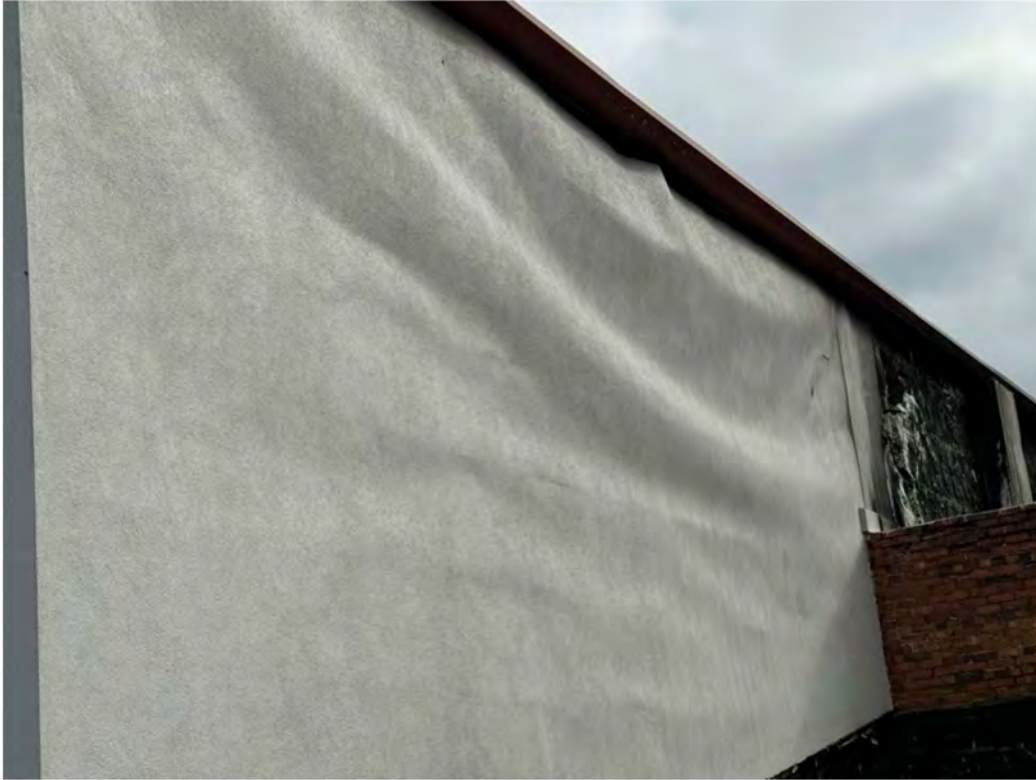
7. Melted fiberglass reinforced plaster siding.
