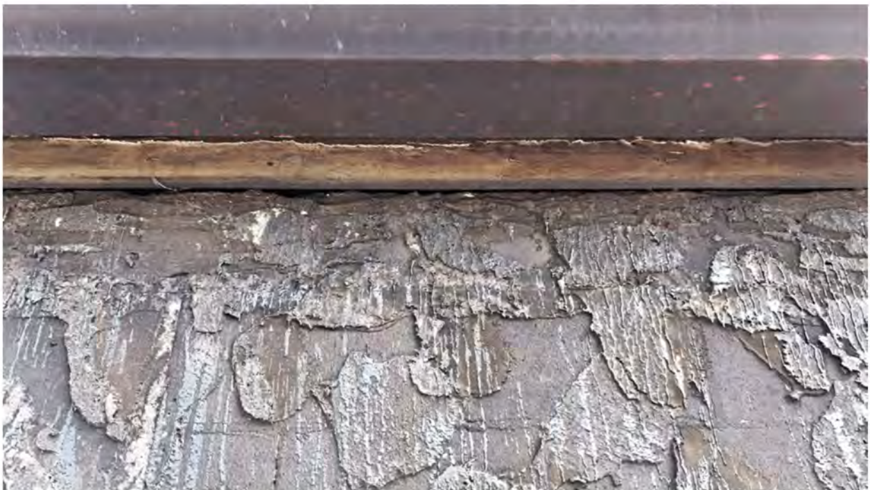
44. Wood sub-facia member below the gutter.
