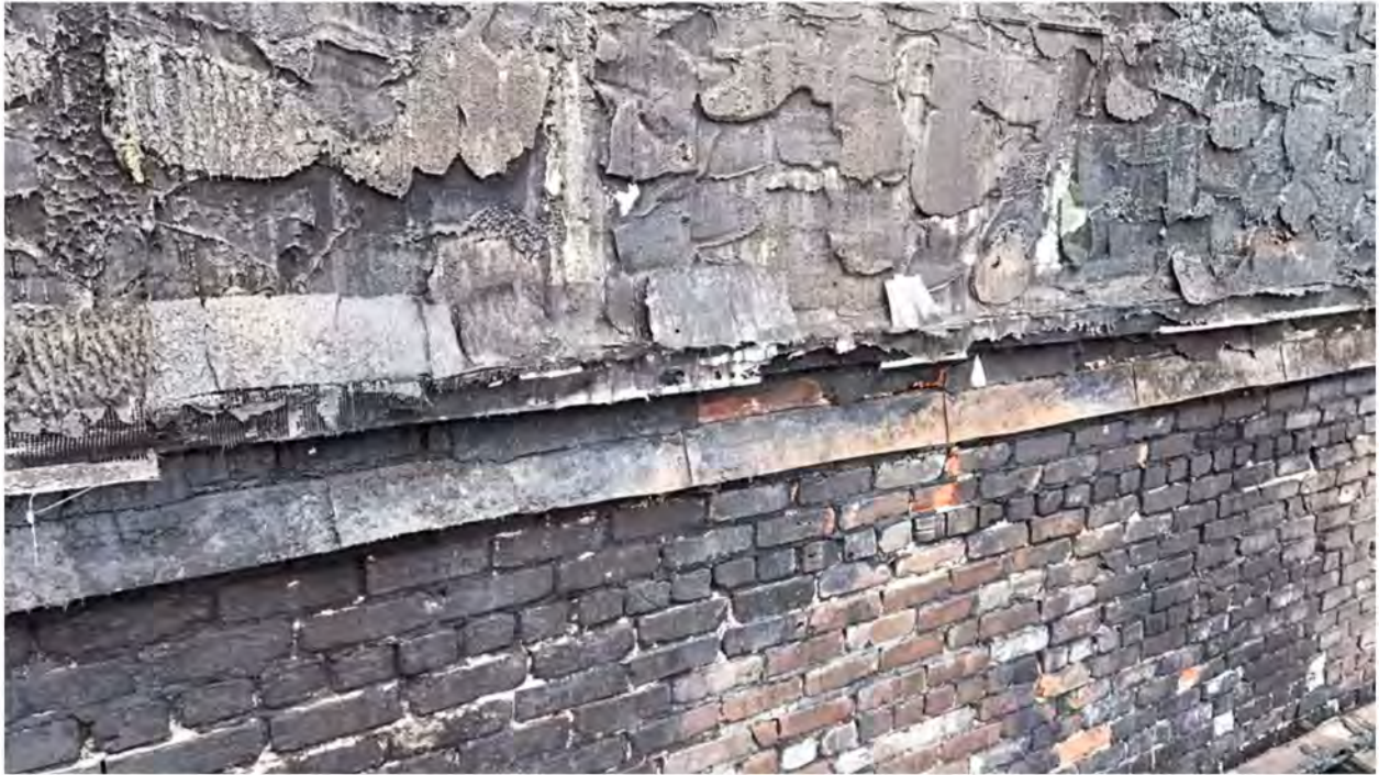
47. Flashing between the first and second floor.
