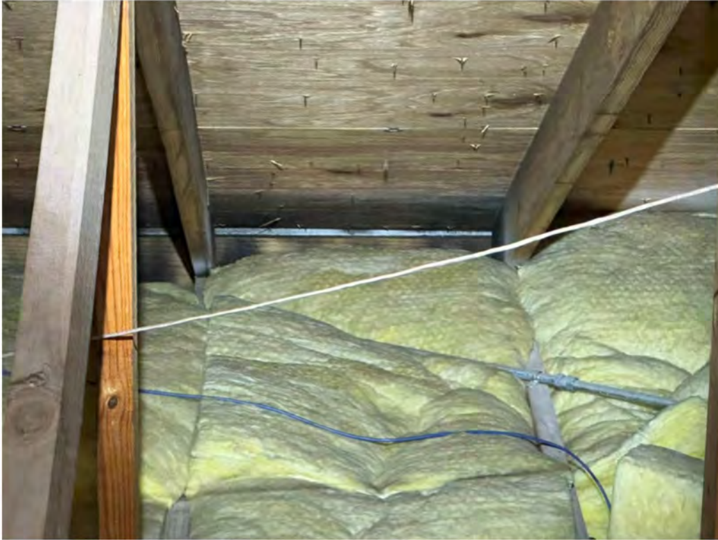
75. Soot accumulation above the western wall.
