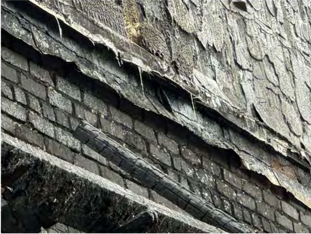
15. Flashing from the adjacent building.
