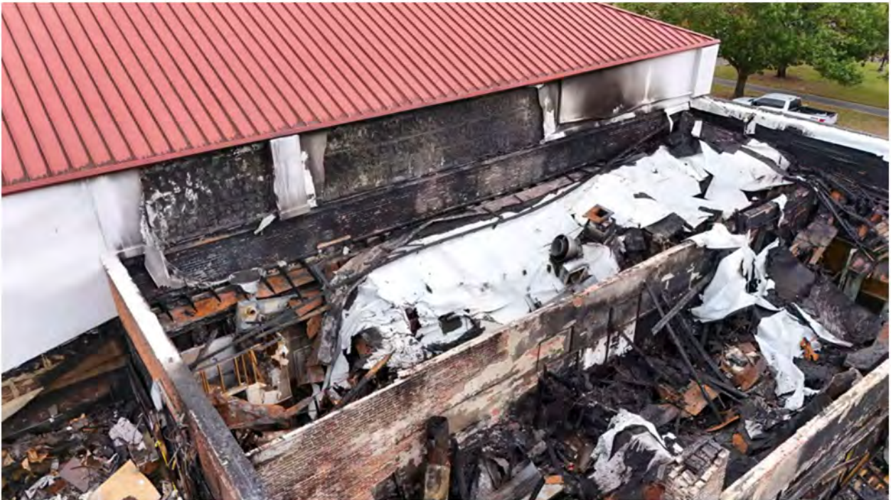
28. Missing siding and exposed masonry walls.
