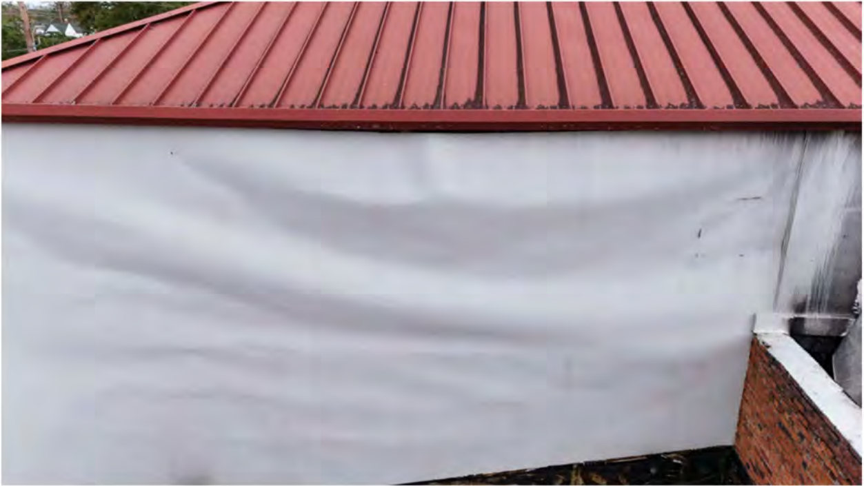
27. Melted reinforced plaster siding.
