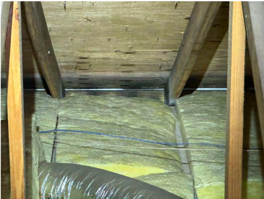
76. Soot accumulation above the western wall.
