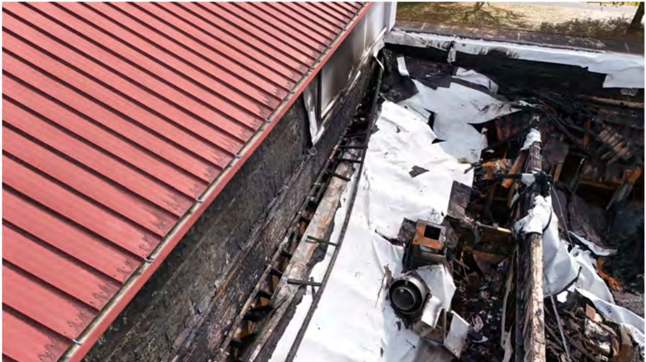
38. Deformed gutter.
