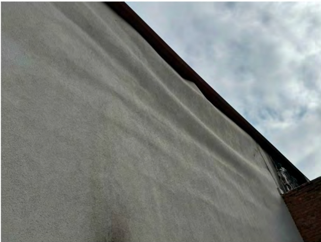
8. Melted fiberglass reinforced plaster siding.
