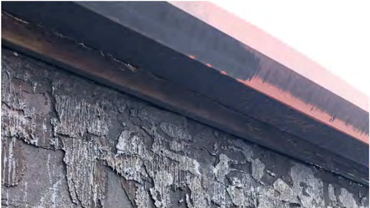
36. Wood sub-facia member below the gutter.
