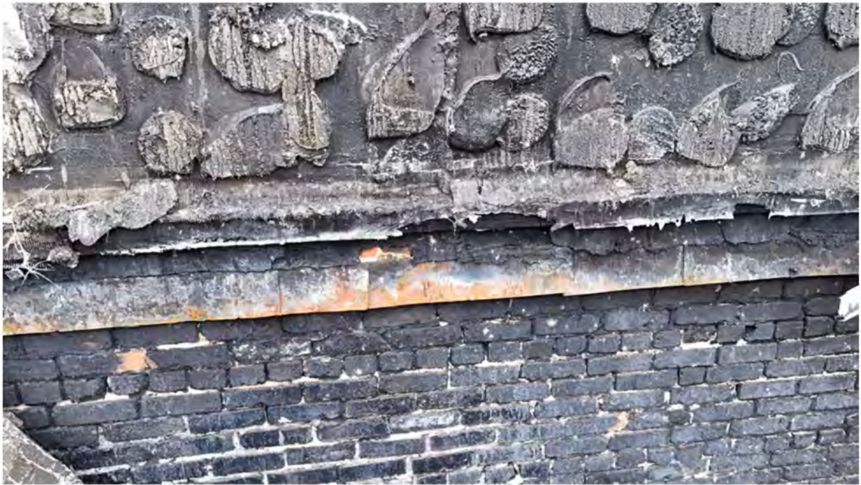
51. Flashing between the first and second floor.
