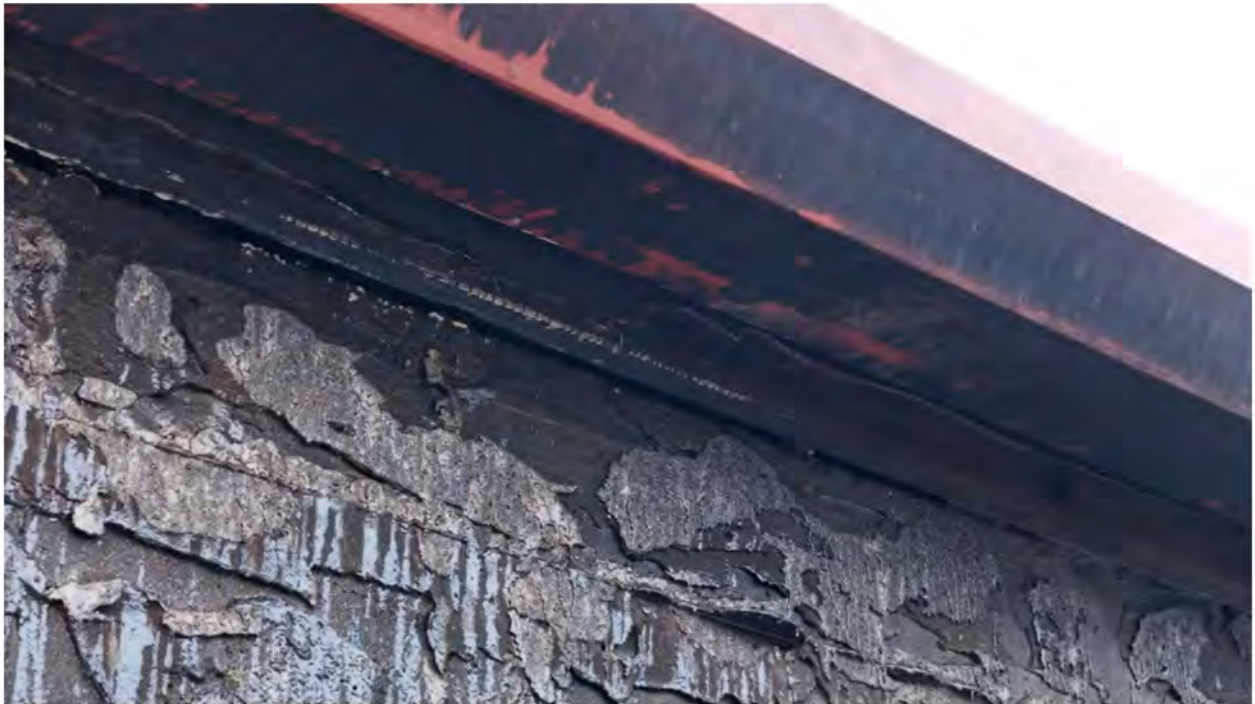
42. Wood sub-facia member below the gutter.
