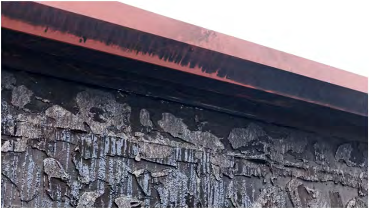
39. Deformed gutter.
