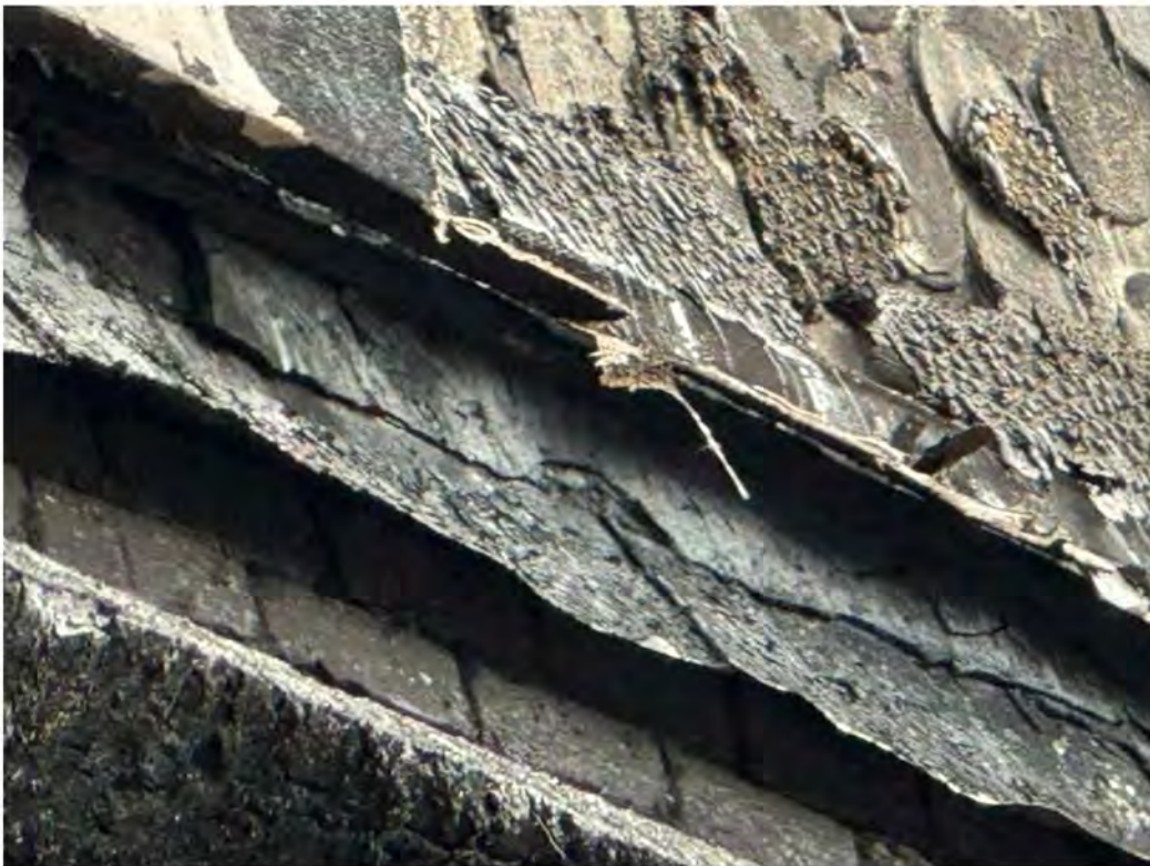
16. Flashing from the adjacent building.
