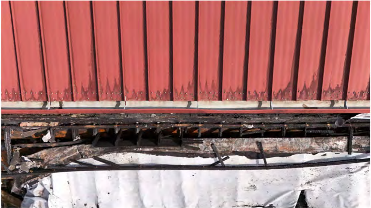
37. Deformed gutter.
